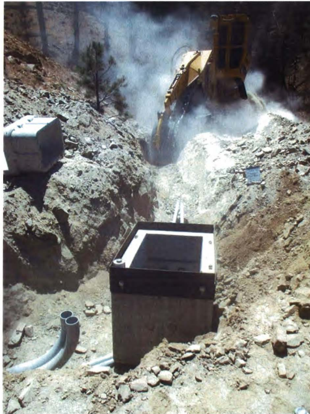
Figure 21 - Installation of underground fiber optic cables in the upper Santa Fe watershed
